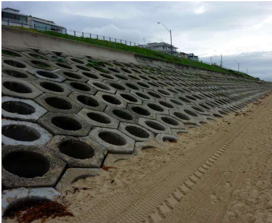
Figure 12 Pre-cast Concrete Revetment
