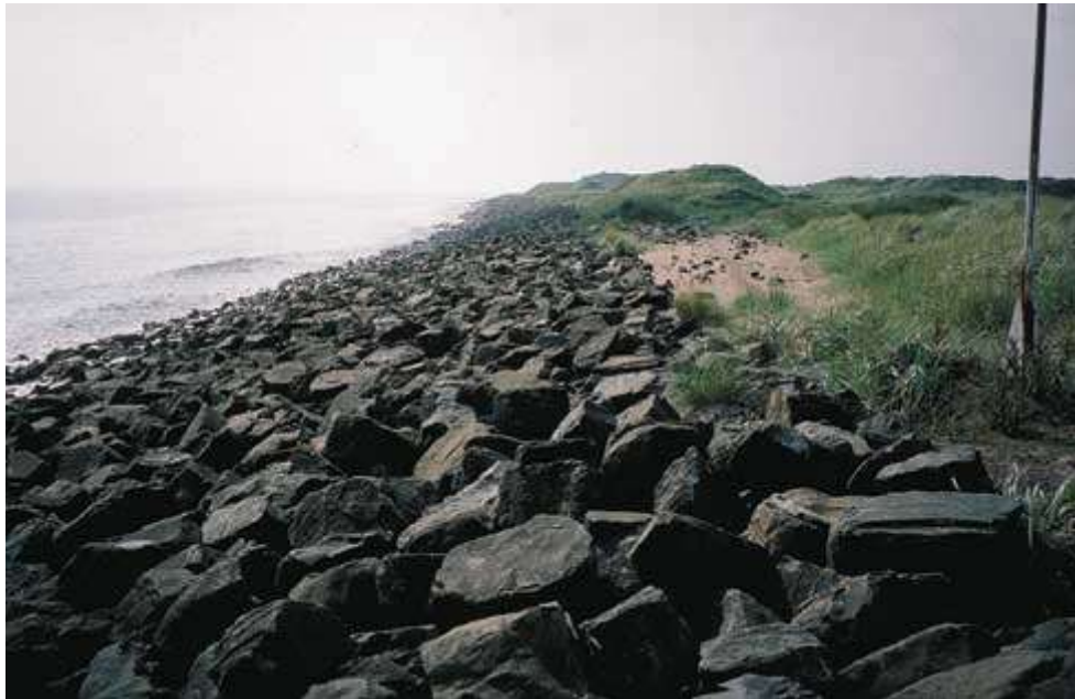
Figure 11 Rock Armour Revetment
