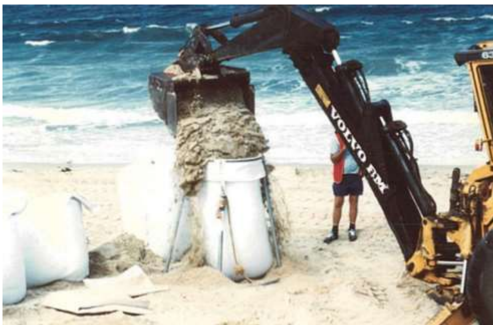
Figure 13 Filling geo-textile containers
