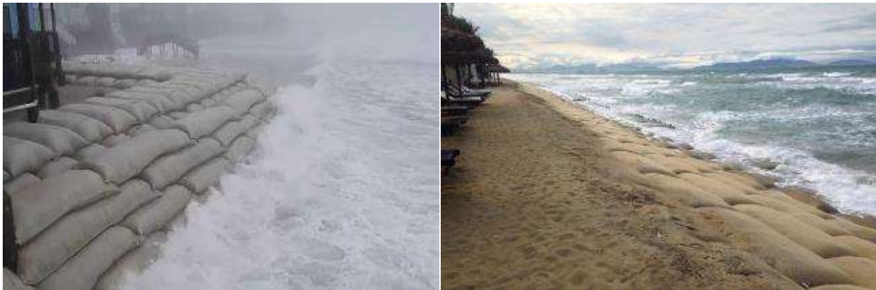
Figure 14 Use of geo-textile containers in high wave energy environments
